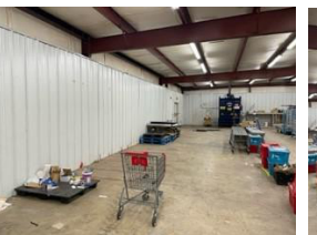
DEMO EXISTING METAL LINER PANELS, LIGHTING, HVAC IN BACK OF HOUSE
