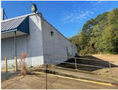
DEMO EXISTING RAMP AND HANDRAIL NEW CONCRETE STEPS AND RAILINGS
